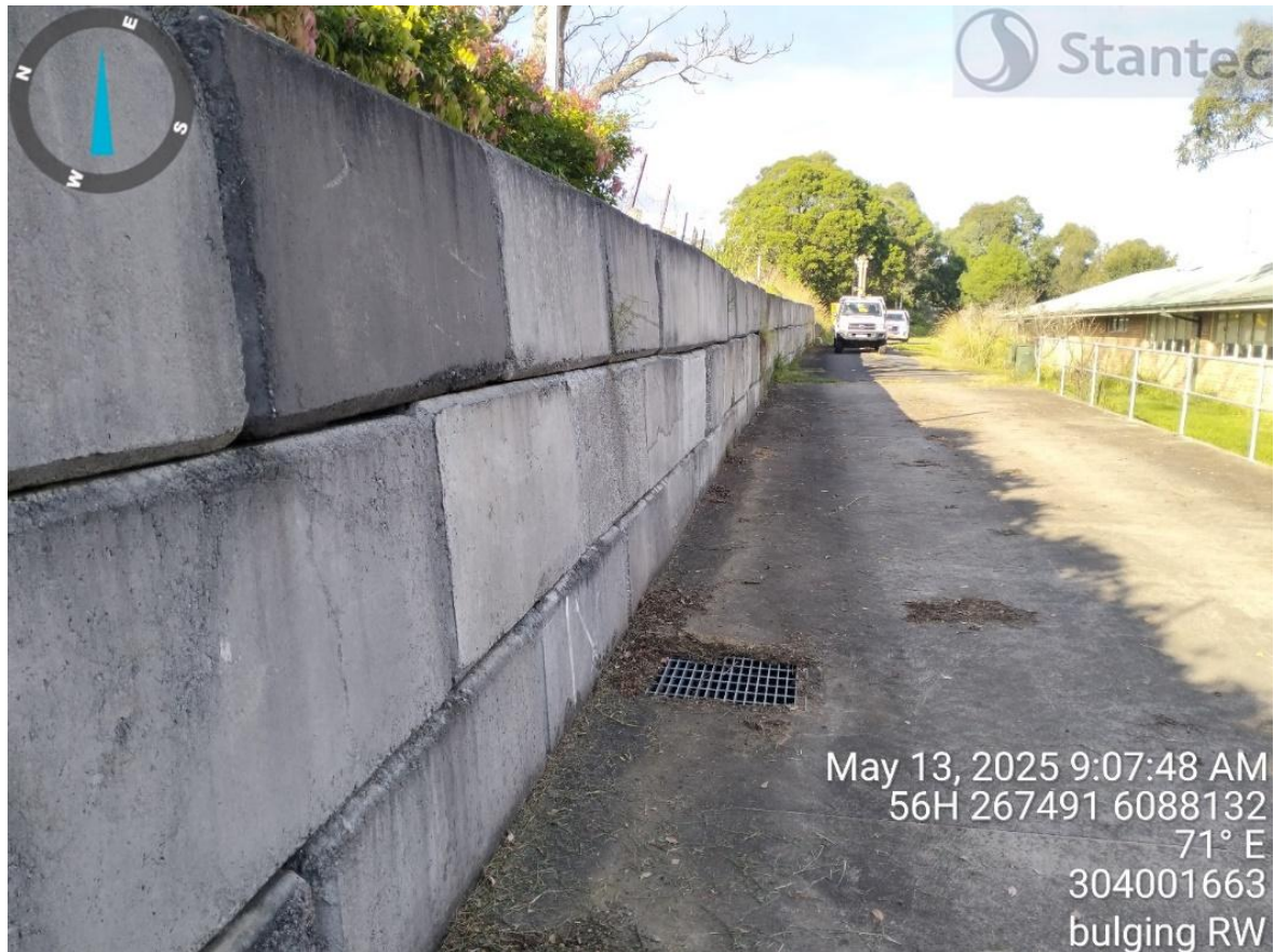
Figure 5-1: Concrete Block Retaining Wall
